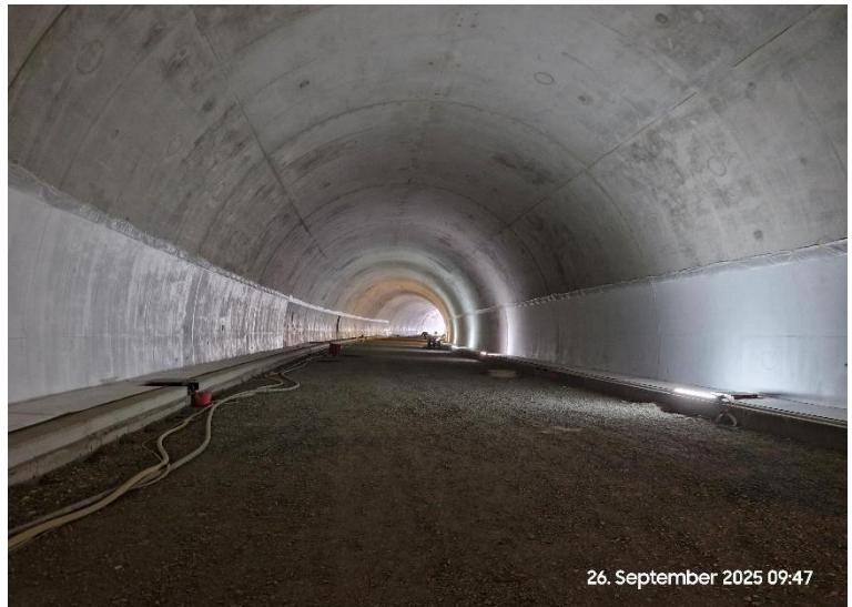
Blick in den fast fertigen Tunnel
